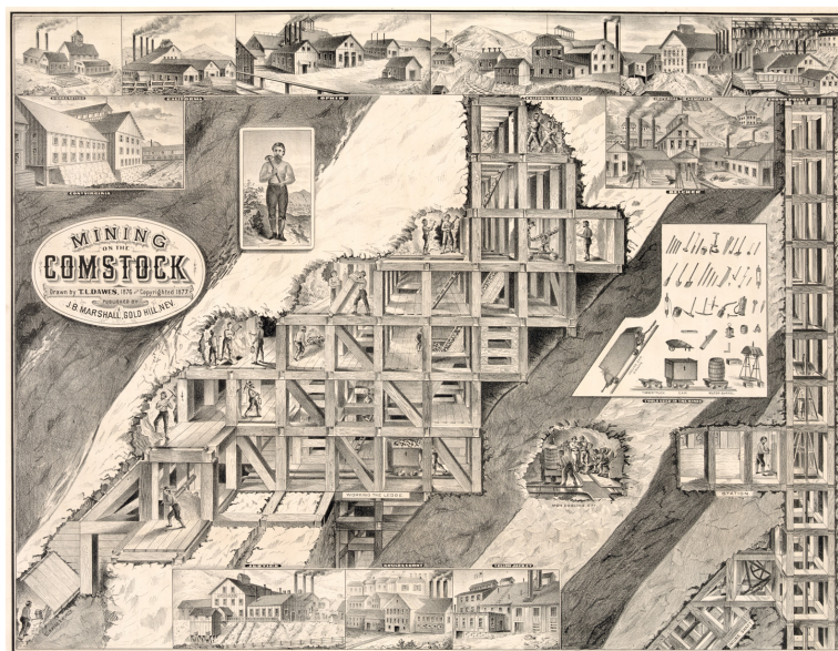
Mining on the Comstock, a lithograph from 1877 depicting the square-set timbering method first developed in the Comstock mines, the various headframes and mills of mines, mining tools, cooling rooms, and shafts. Drawing by T.L. Dawes; Le Count Bros., Lith., San Francisco.
